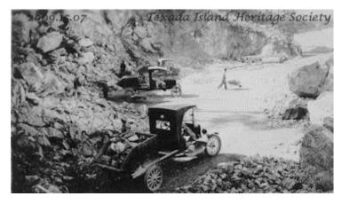
Lime rock was "shot out" of the cliffs, drilled, then broken by hand hammer. The hundred-pound "man-sized rock" was muscled onto the small 1924 Model-T Ford dump truck by the "B&L" (Breaker and Loader) crew. It is reported that Big Joe Little could easily lift and carry even larger pieces.
